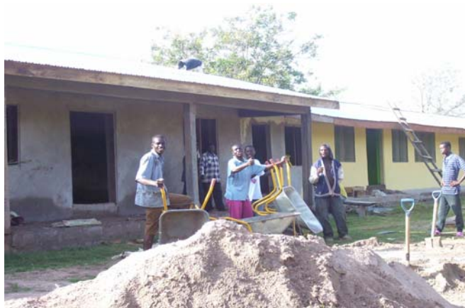
Villagers Building Additional Classrooms
