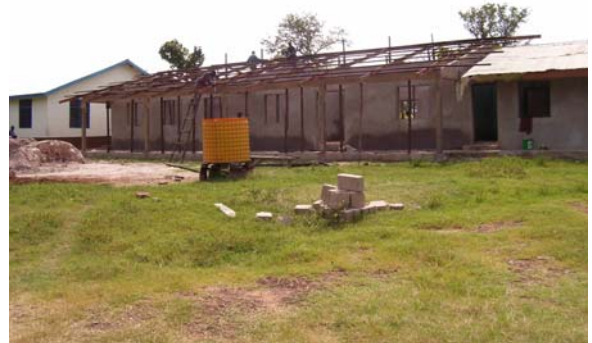
a Villager Roofing Additional Classrooms
